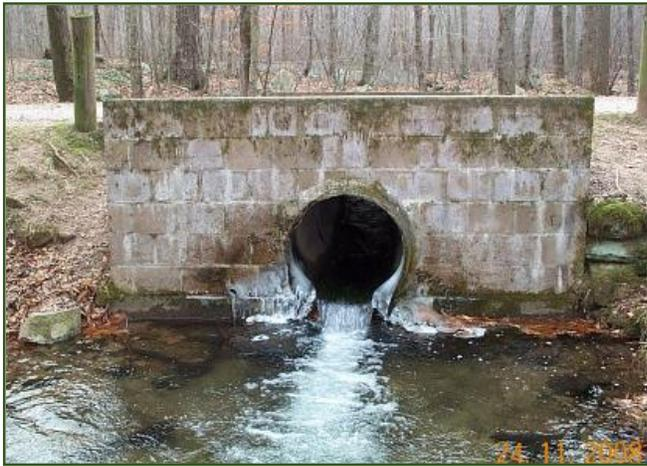
Left. Outlet of 30 inch substandard culvert perched above the Mott Hill Brook streambed that blocks and prevents upstream passage for the wild Brook Trout population.
